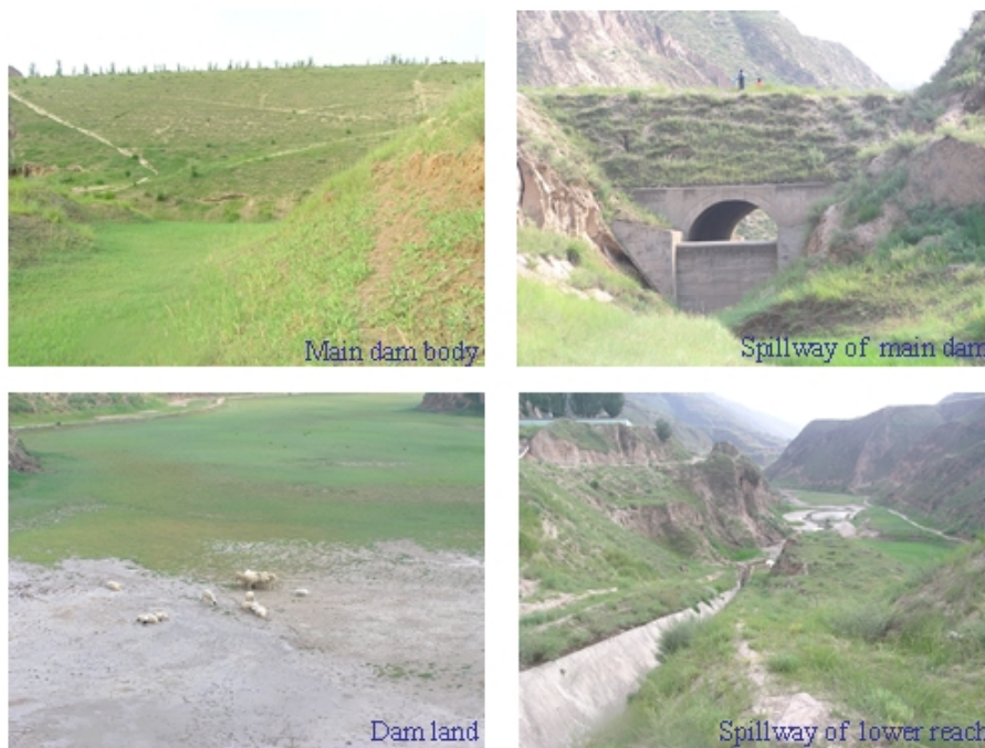
Figure 4.6. Major components of skeleton dam
